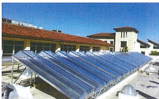
图16 Micro-Concentrator (MCT)集热器运用
